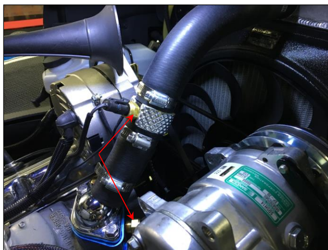
Photo 5: Installation complete. Temp readings at both locations were verified within 2°.
